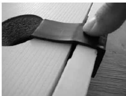
Push Reveal Spacer down into Reveal Lock.
