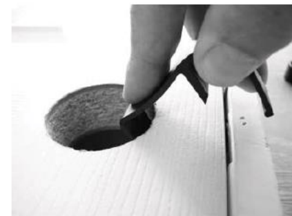
Pull the clip over the face of the door.
