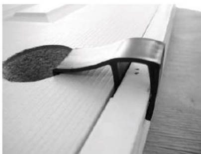
Pull jamb secure tab over jamb.
