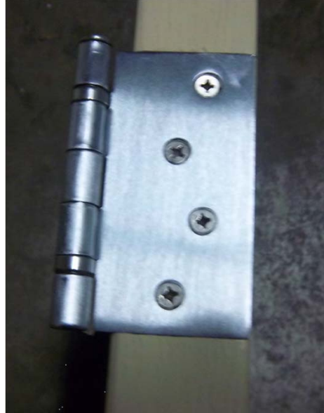
Aribell's 4 1/4" x 4" Fiberglass Door Hinge No "Gap".
